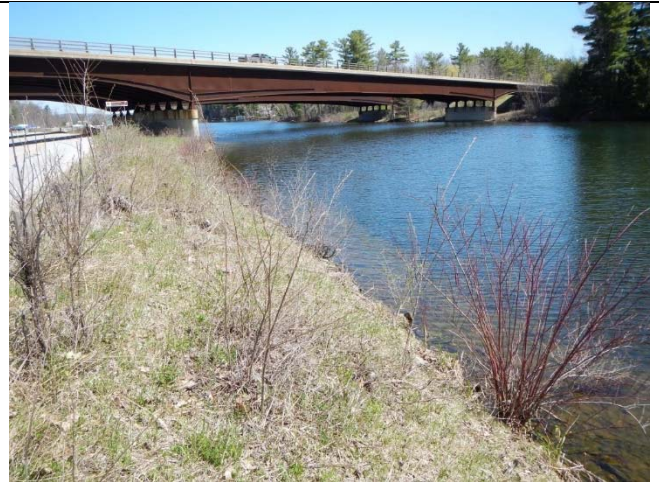
Photograph 14. Bridge on U.S. 4, over Lake Bomoseen, V-LB-OHW-1, in Fair Haven, VT
