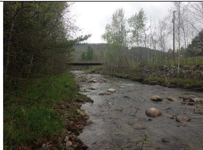
Photograph 34. View of local network and bridge over T-LU-S-2 in Ludlow, VT
