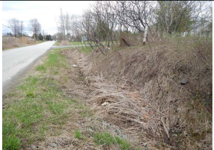
Photograph 12. Road and residential area, near V-FH-S-2 off of VT 22A in Fair Haven, VT
