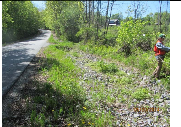
Photograph 8. Hullet Hill Road in Benson, VT
